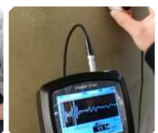
FRP Oil Tank
